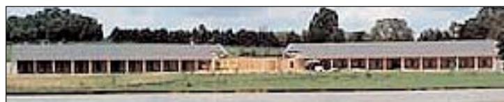
The Rivive Us Again Retreat Center in Dittmer, Mo., is under construction this summer. The main meeting hall is shown at top. The sleeping rooms, below. The center will accommodate 164 people.
